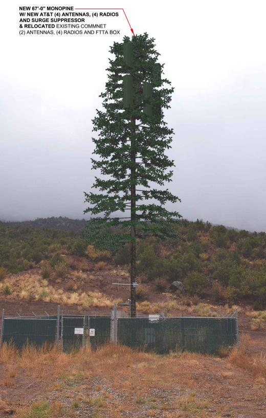
DISCLAIMER: THIS PHOTOSIMULATION IS INTENDED AS A GRAPHICAL REPRESENTATION OF EXISTING AND PROPOSED SITE CONDITIONS BASED ON THE PROJECT / DRAWING PLANS. IT IS NOT INTENDED FOR CONSTRUCTION. ACTUAL, FINAL CONSTRUCTION MAY VARY
